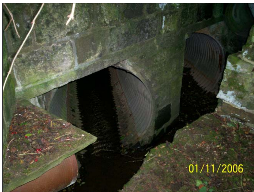
Entrance to Carlton Bramhope highway culvert
