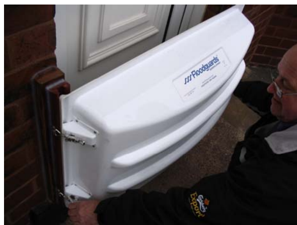
Installation of a door flood guard
