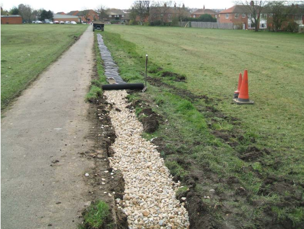
New land drain being installed at Stanningley Park
